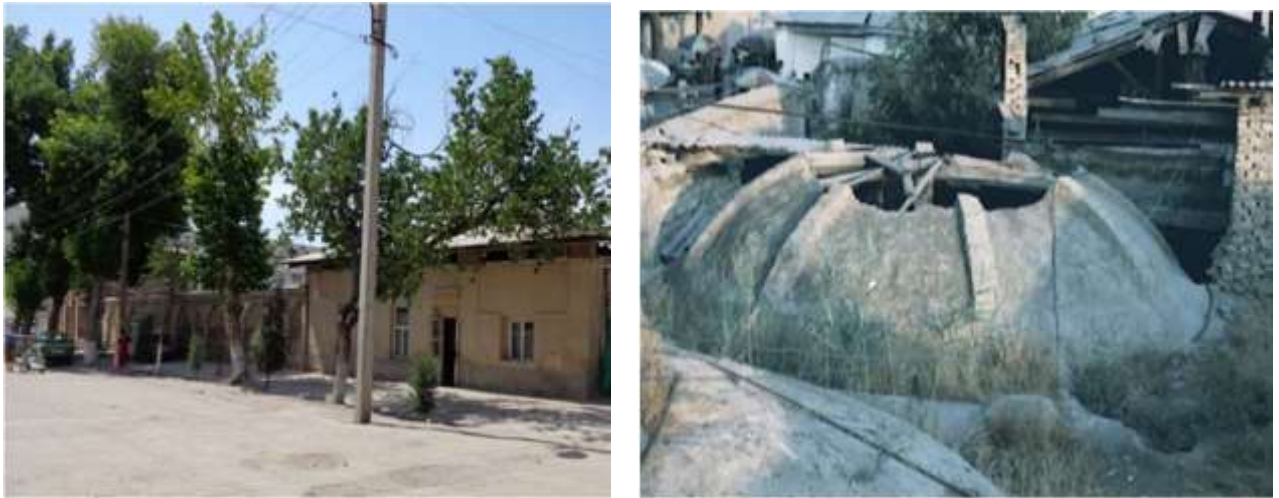
Figure 3. General view of Latif's bathroom.3-пачм.
